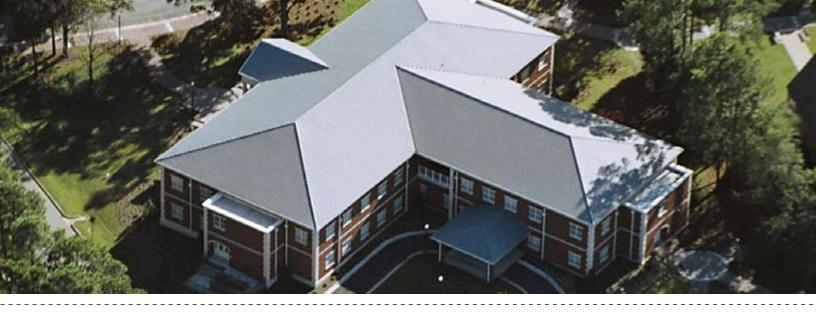
This revolutionary coating system consists of PVDF resin, acrylic resin and pigments, which give the product its incredible color, durability (fade resistance), and energy efficient "coolness." PVDF (Polyvinylidene Fluoride) is a highly non-reactive and pure thermoplastic fluoropolymer. It is also known as KYNAR 500°, a registered trademark of Arkema, Inc. or Hylar 5000°, a registered trademark of Solvay Solexis.
